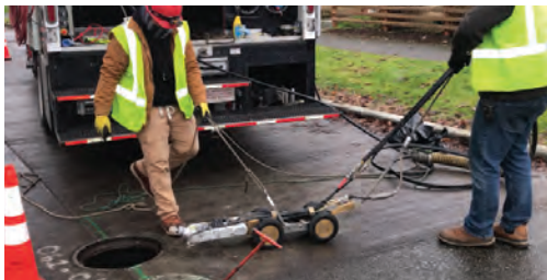
SEATTLE PUBLIC UTILITIES 2020—IN PROGRESS SEATTLE, WA
