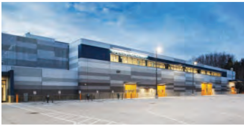
SOUND TRANSIT 2017—IN PROGRESS BELLEVUE, WA
